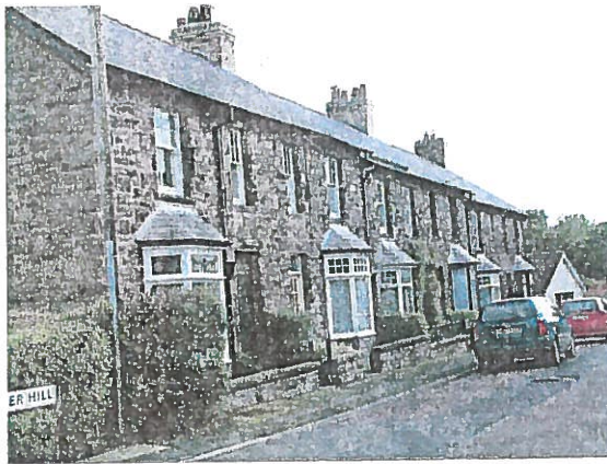
Rock faced stone finish on cottages on Tenter Hill
