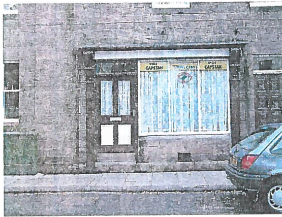
An attractive modest Victorian shop front
