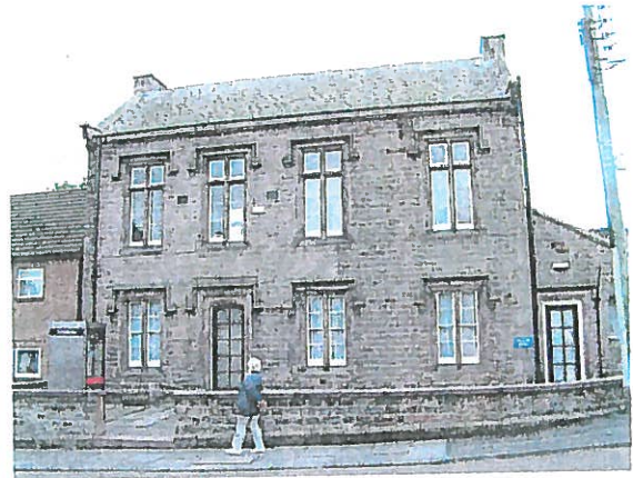
Carved hood moulds on Old Register Office 1859. These are a distinctive feature in Wooler
