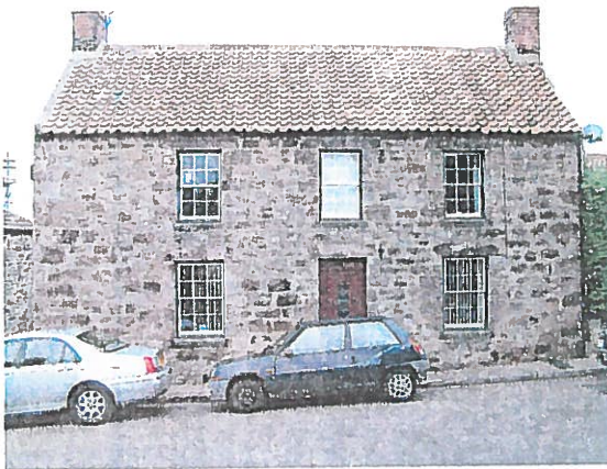
A buttering of mortar over stone arrises.
