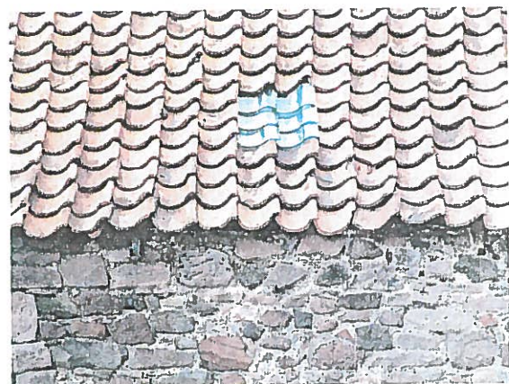
A pantile roof with pantile shaped glazing.
