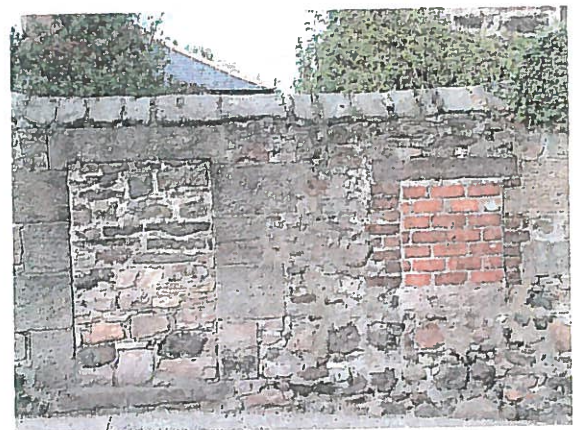
Blocked in openings in boundary wall.
